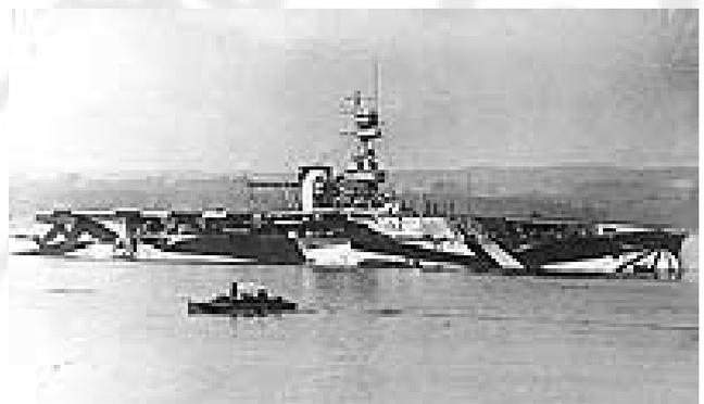
HMS Furious. Note fly-off deck forward and landing on deck aft.
